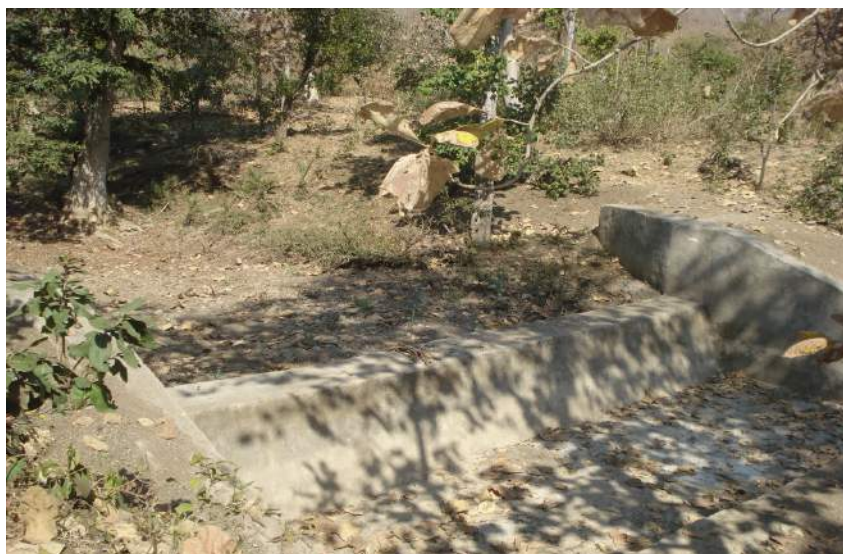
Check dam - Comptt. no.10, Beat- Kosdani, Range– Ami
